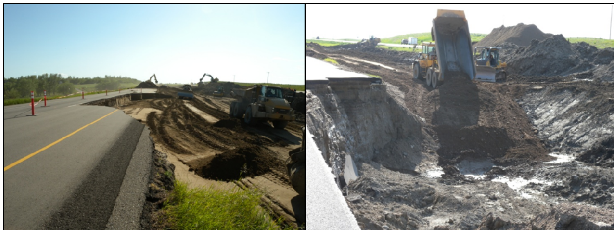
Figure 4 – Placing granular material.
