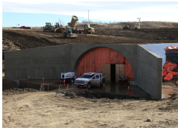
Figure 8 – Geosynthetically confined soil wall behind wingwall.
