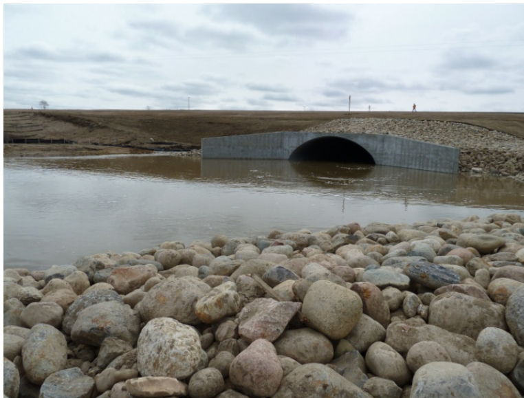
Figure 11 – Completed culvert and riprap December 2010.
