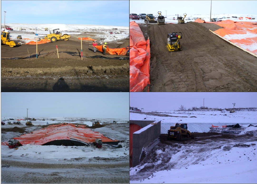
Figure 7 – Backfilling granular material in winter conditions.
