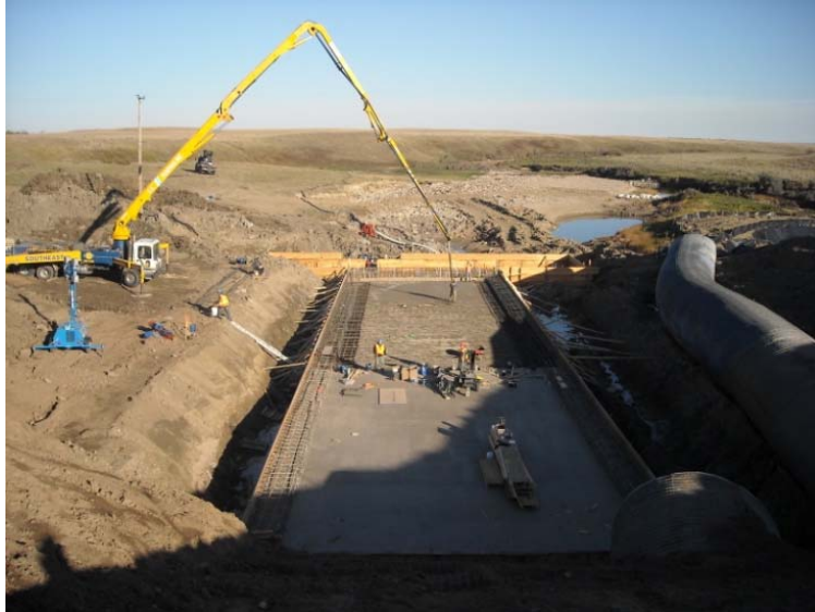
Figure 5 – Concrete pour for raft slab foundation.
