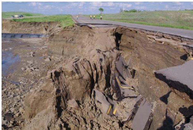
Figure 2 – Remaining eastbound lanes, looking east.
